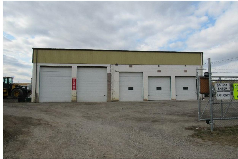
Photo #A2: Gravel paved driveway.
