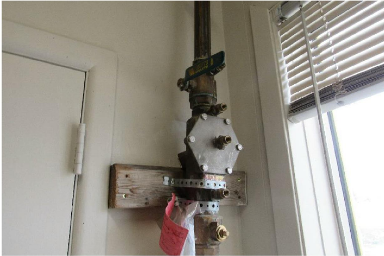
Photo #M5: Backflow prevention device in the washroom area of the Main Shop.
