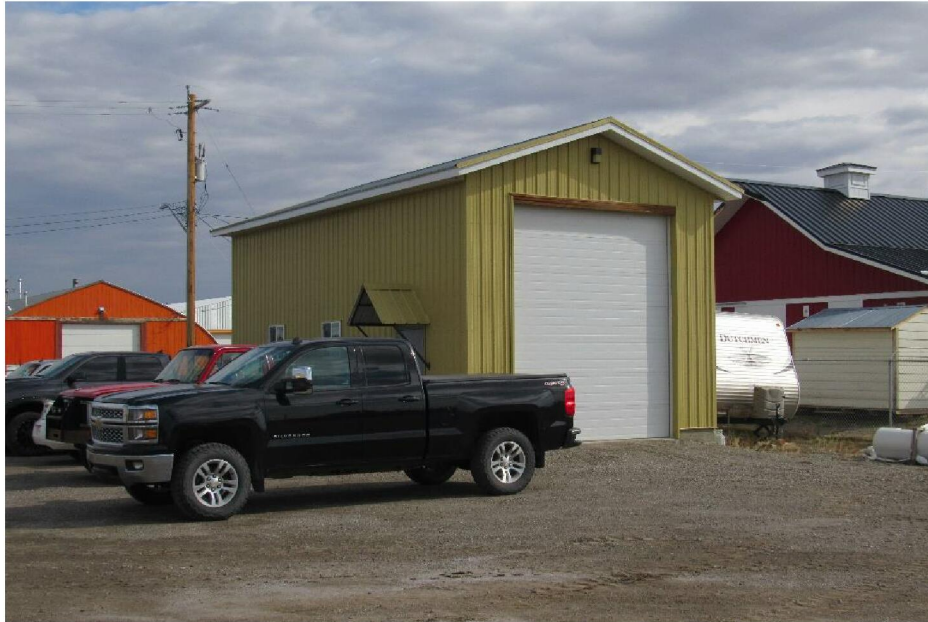
General view of the East Shop.
