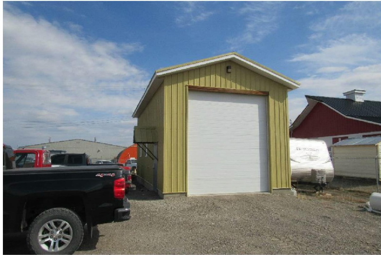
Photo #A5: General view of the East Shop.
