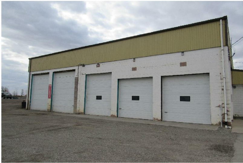
Photo #A3: General view of the Main Shop.
