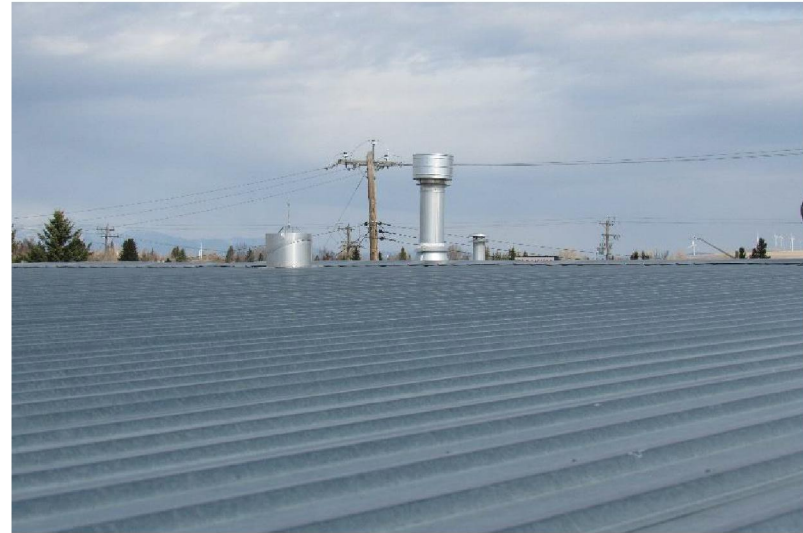
Photo #A14: General view of the Main Shop roof.
