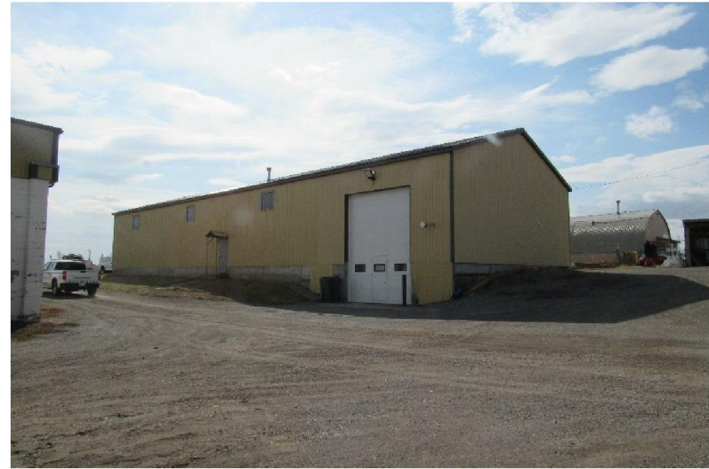
Photo #A4: General view of the South Shop.
