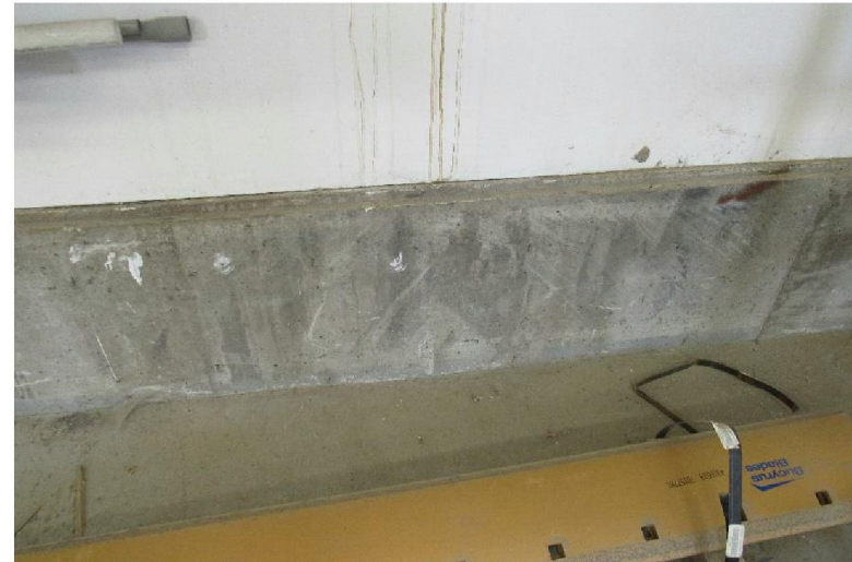
Photo #S2: Exposed the South Shop CIP foundation wall.
