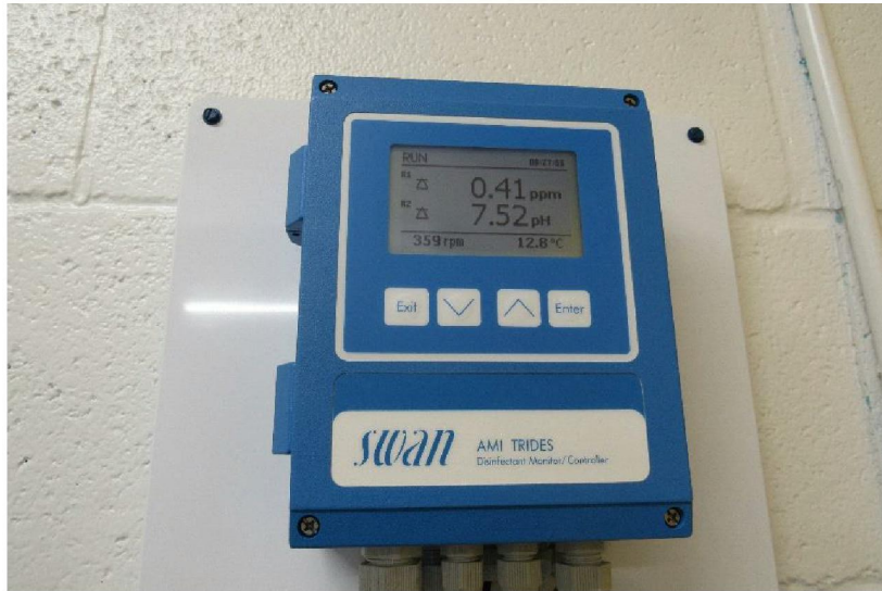
Photo #E5: Carbon monoxide detector in the Main Shop.
