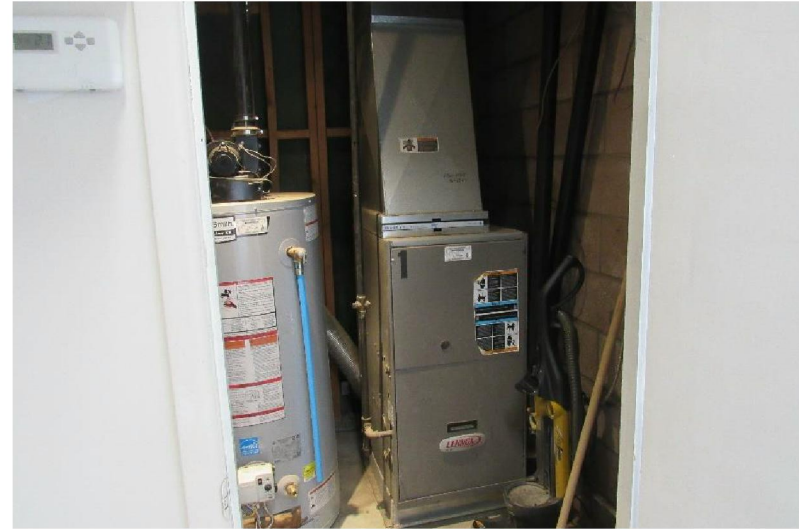
Photo #M6: One (1) gas-fired water heater alongside a furnace, in the mechanical room of the Main Shop.
