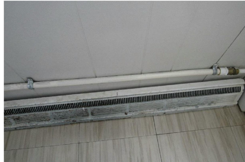
Photo #M8: Typical baseboard found in the Main Shop washroom area.
